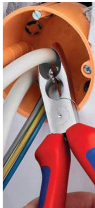
Stripping deep down in a flush-mounted junction box
